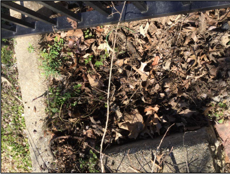
Photo 13: View of outfall 11 in.
