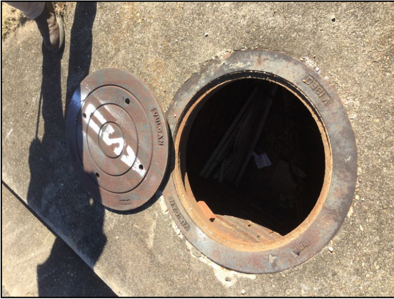
Photo 25: View of outfall 17 in.
