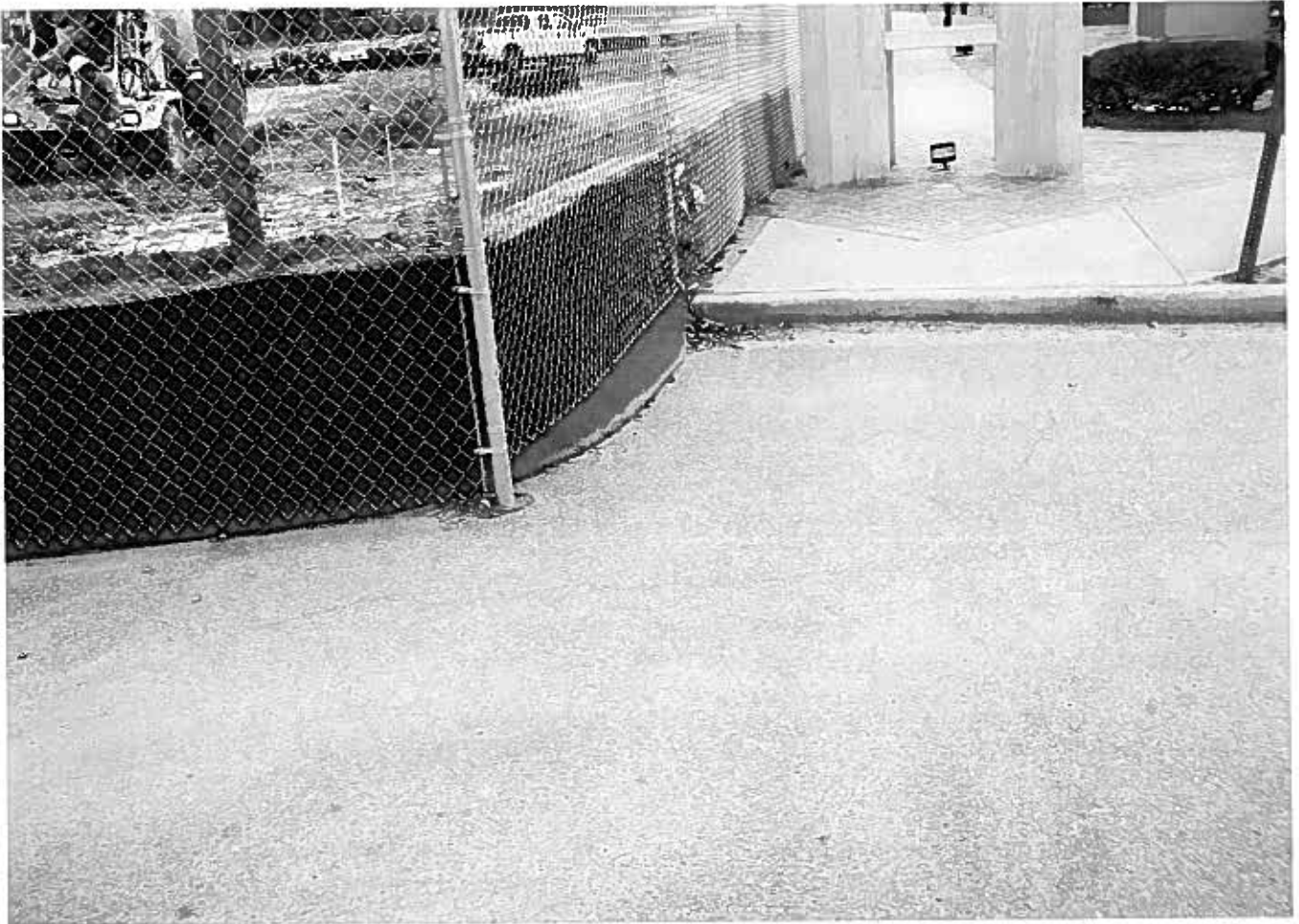
LIBRARY - CLEAN SILT FENCE
