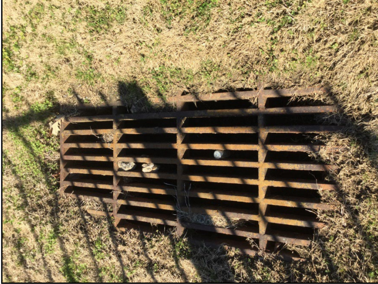
Photo 5: View of outfall 7 in.
