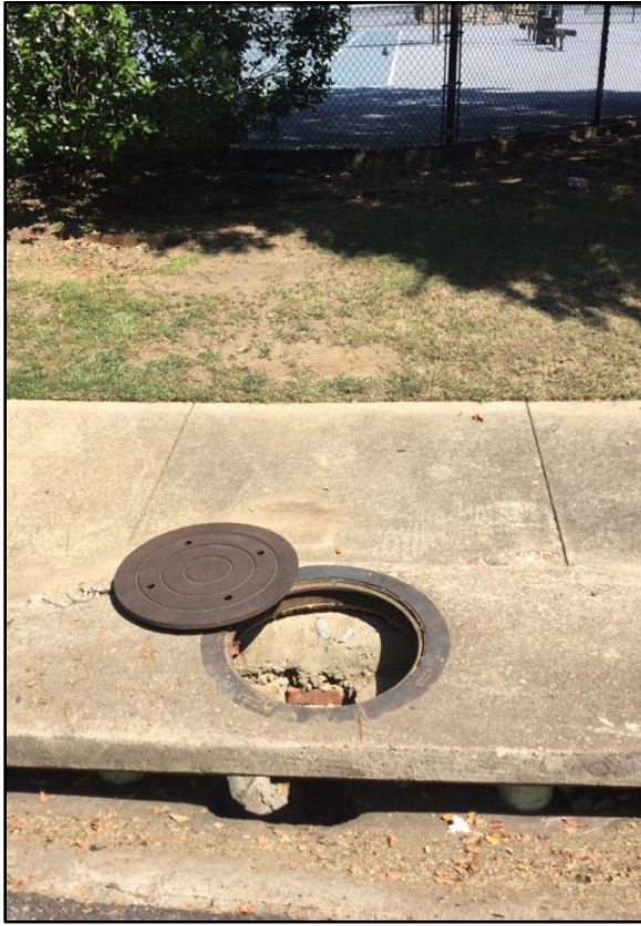
Photo 15: View of outfall 12 in.
