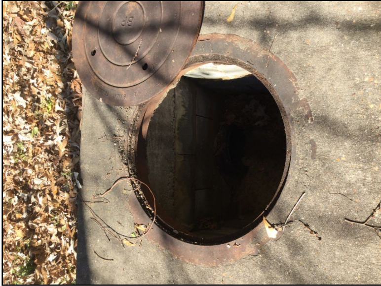
Photo 27: View of outfall 18 in.
