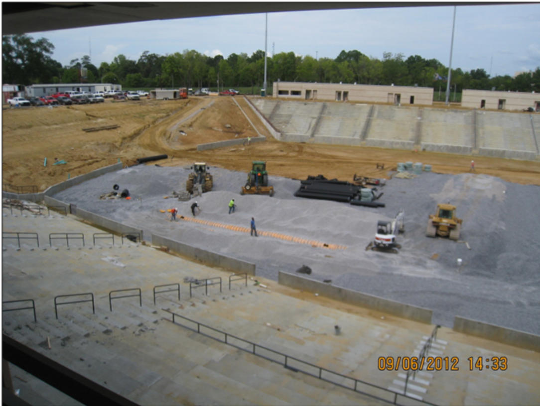
Football Stadium Subsurface Stormwater Detention under Construction
