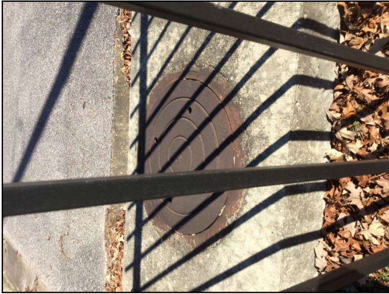
Photo 7: View of outfall 8 in.
