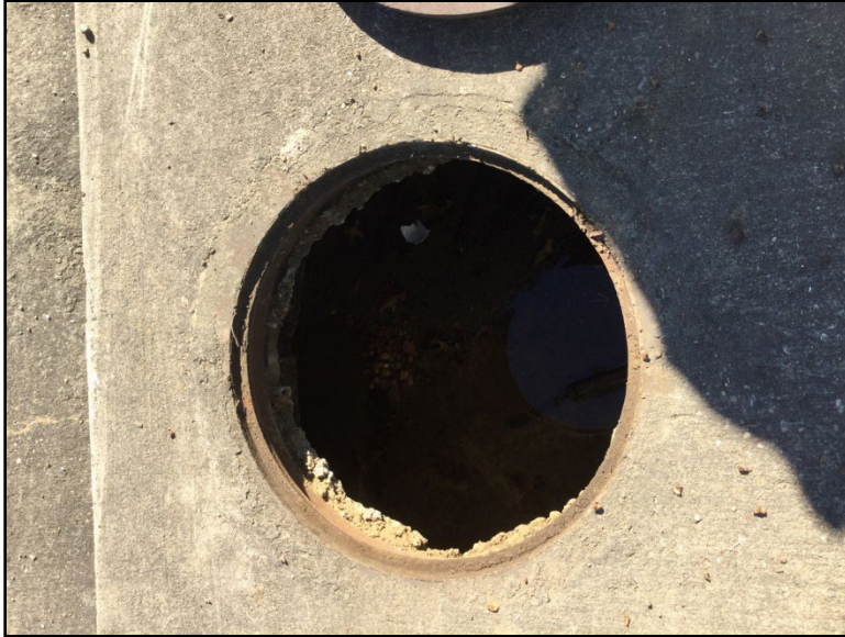
Photo 3: View of outfall 6 in.
