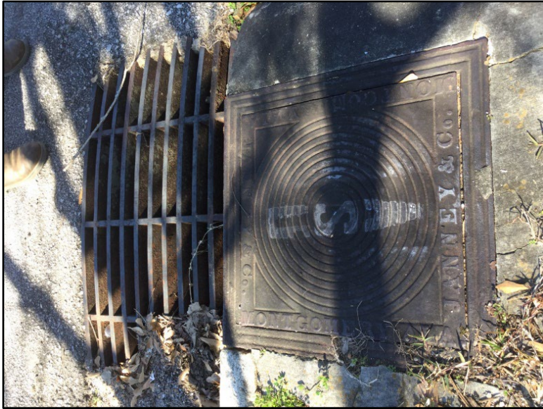
Photo 23: View of outfall 16 in.
