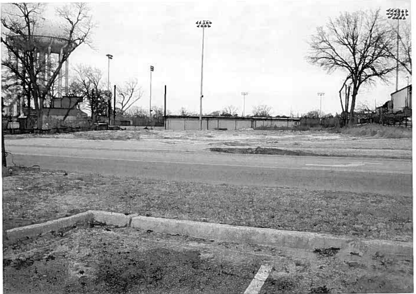
CARTER HILL RD - INSTALL BMP'S
