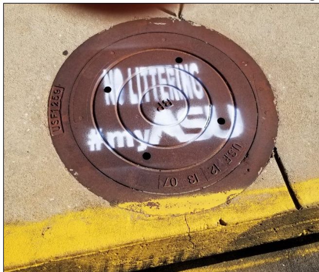
Figure 1. Example of ASU's storm drain marking
