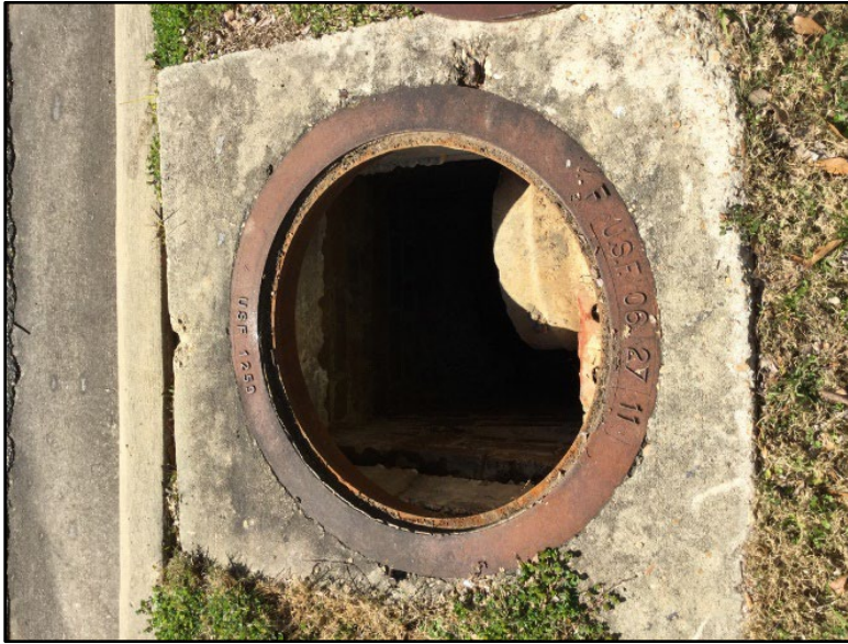
Photo 11: View of outfall 10 in.
