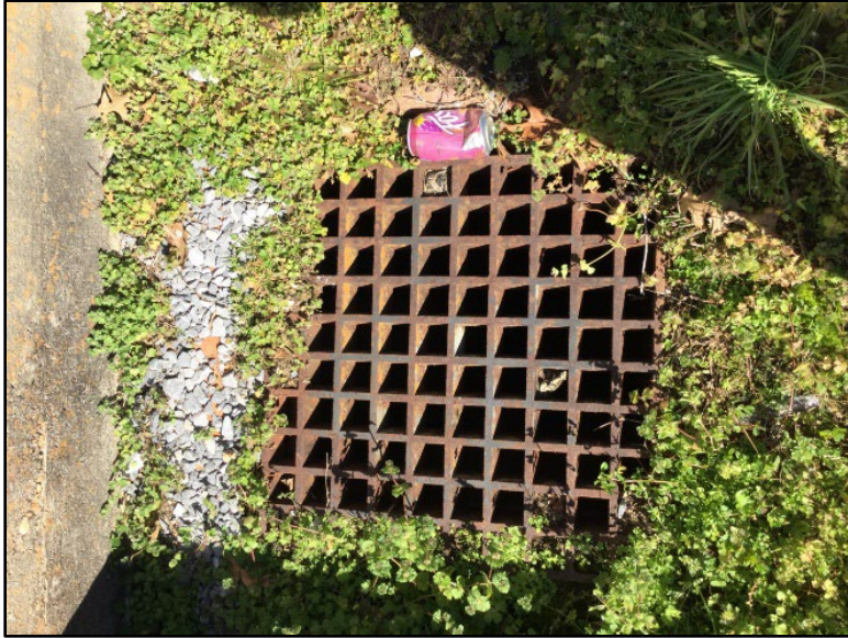
Photo 19: View of outfall 14 in.
