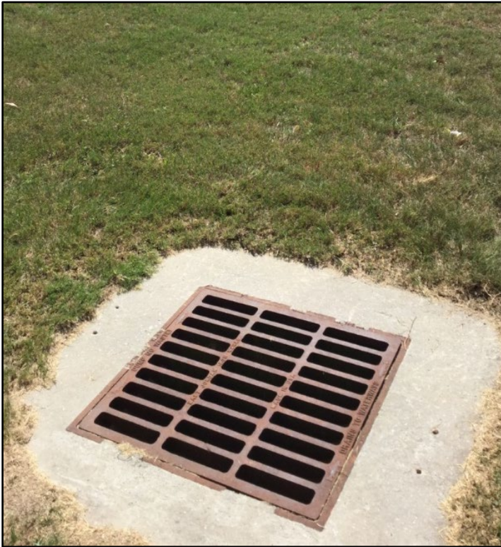
Photo 21: View of outfall 15 in.
