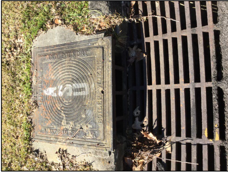
Photo 17: View of outfall 13 in.
