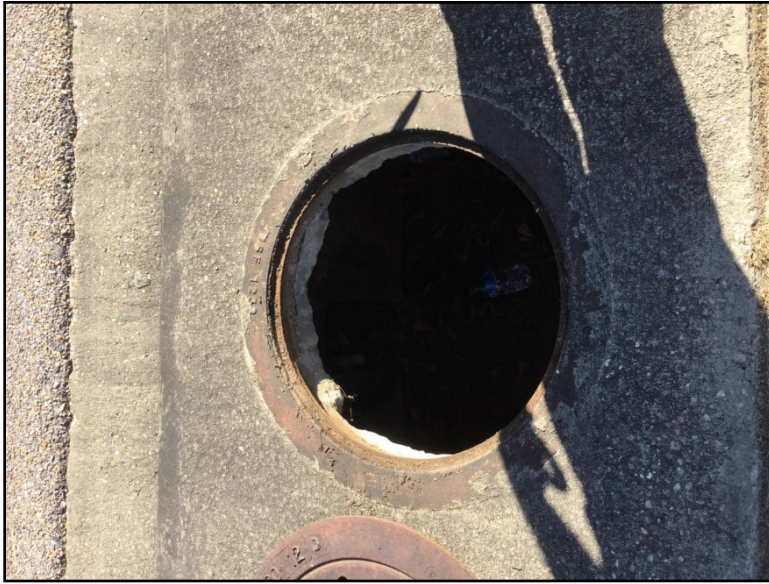
Photo 1: View of outfall 5 in.
