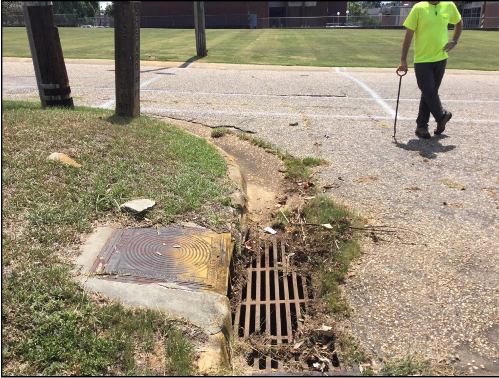
Photo 25: View of outfall 17 in.
