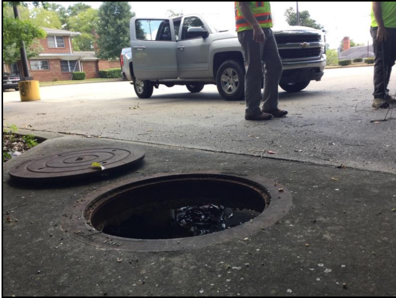
Photo 27: View of outfall 18 in.
