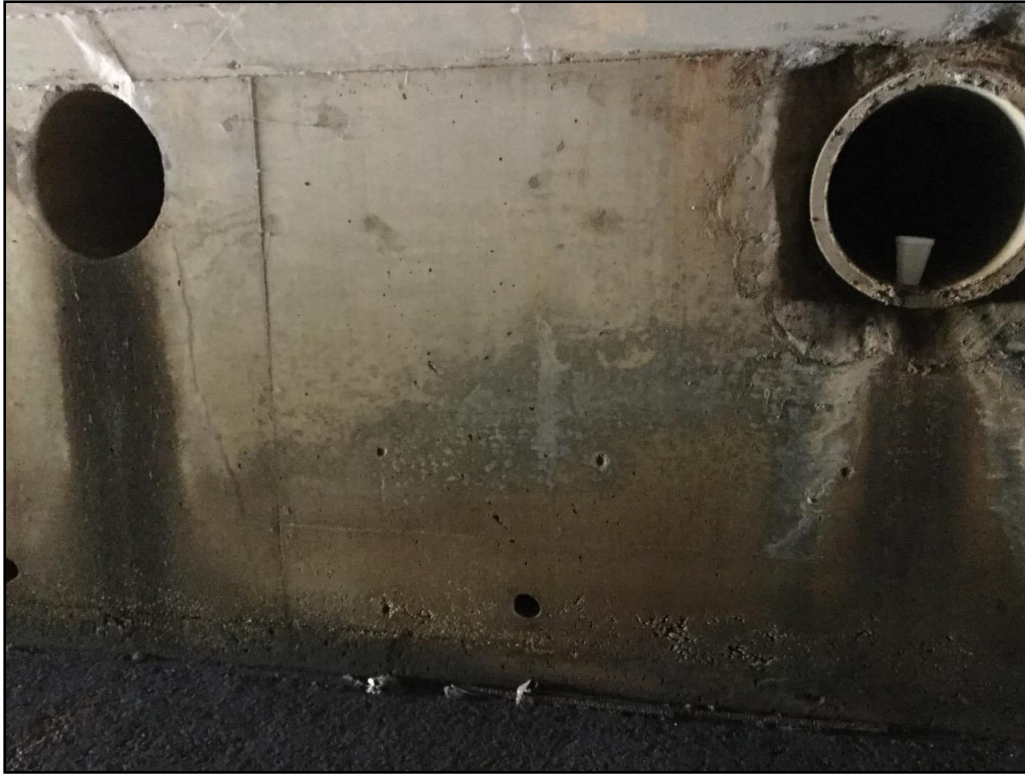
Photo 23: View of outfall 16 in.
