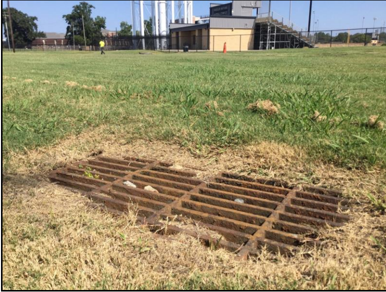
Photo 5: View of outfall 7 in.
