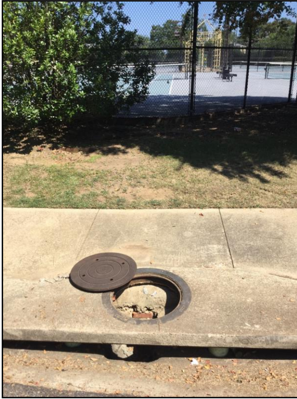
Photo 15: View of outfall 12 in.
