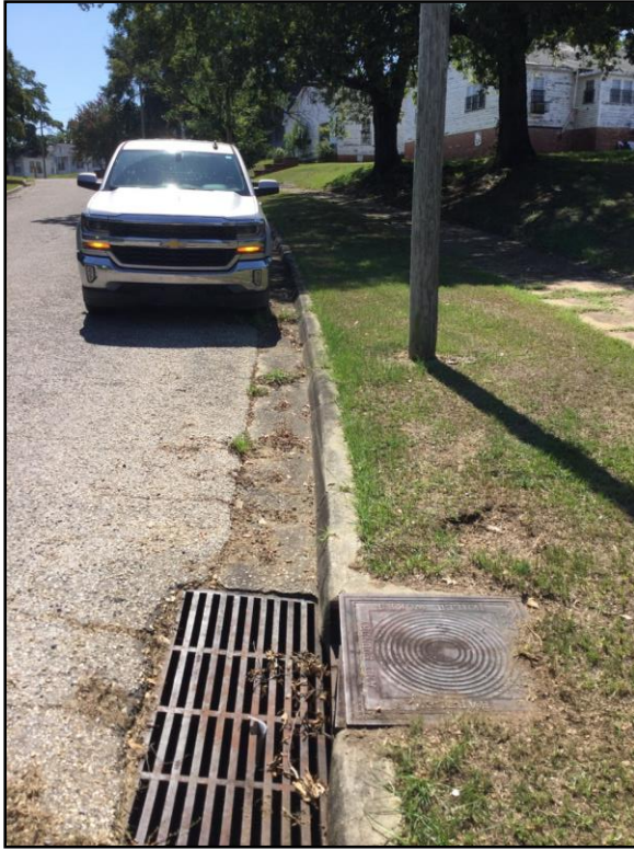
Photo 17: View of outfall 13 in.
