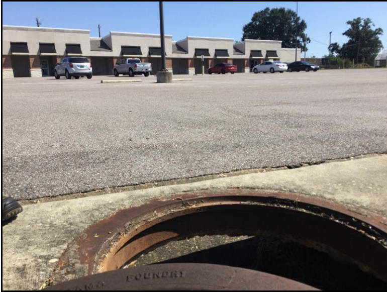
Photo 7: View of outfall 8 in.
