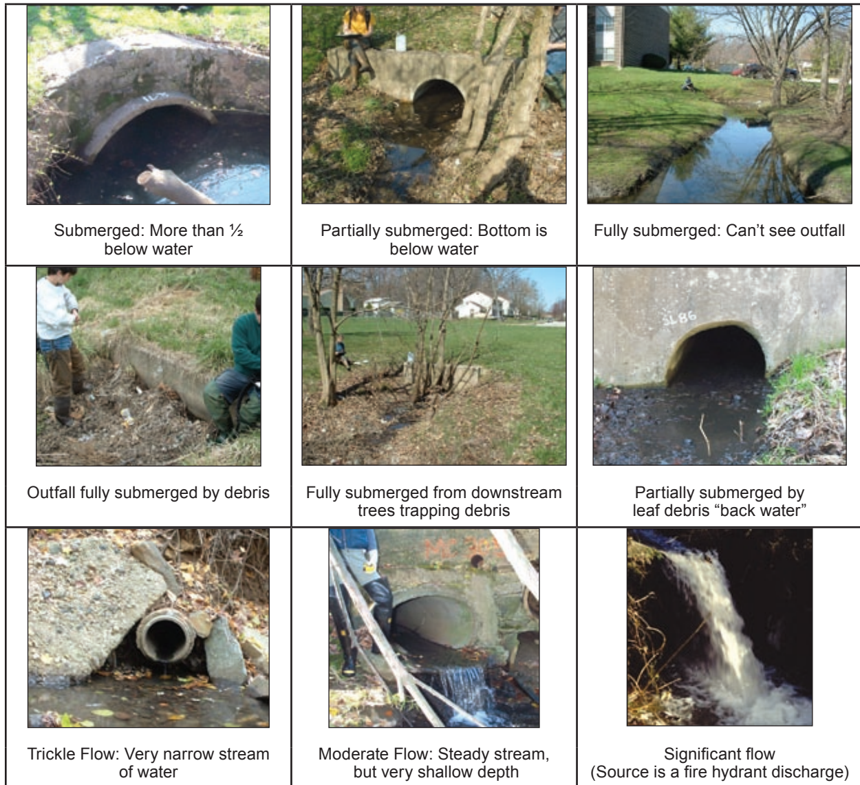
Figure 28: Characterizing Submersion and Flow
