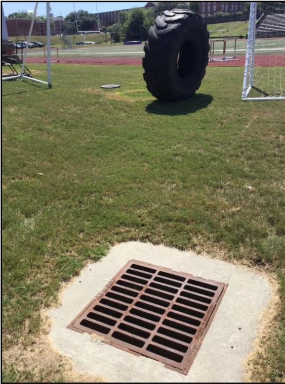
Photo 21: View of outfall 15 in.
