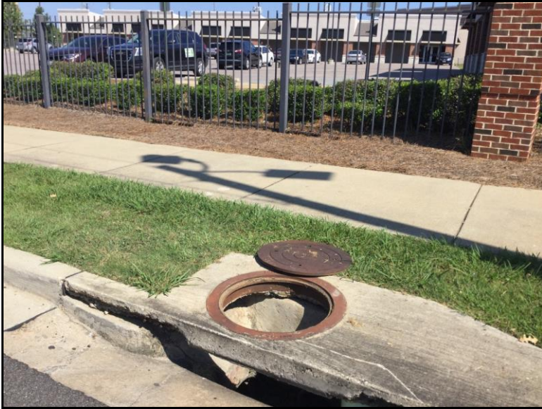
Photo 9: View of outfall 9 in.
