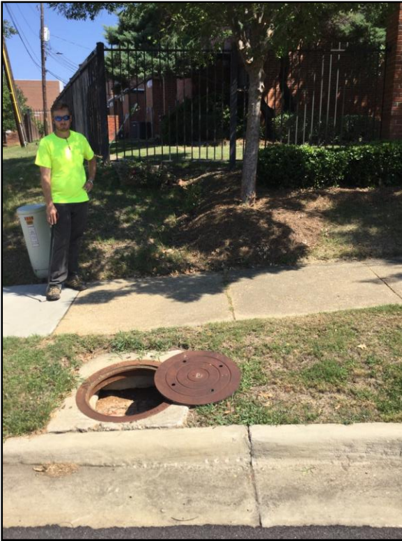
Photo 13: View of outfall 11 in.
