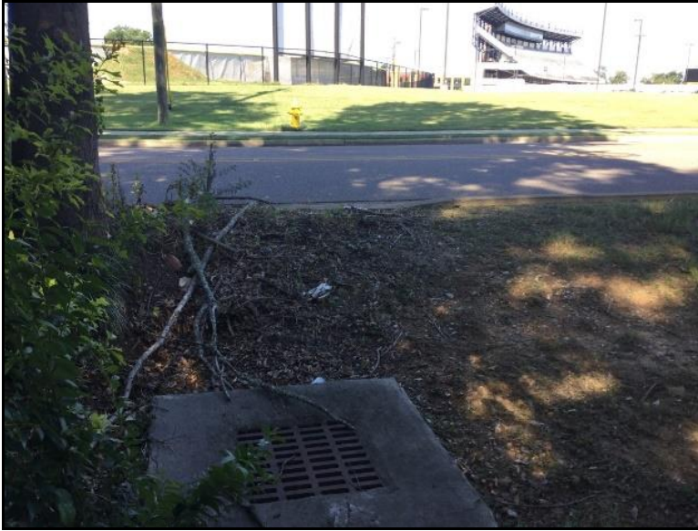
Photo 1: View of outfall 5 in.
