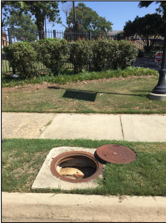
Photo 11: View of outfall 10 in.
